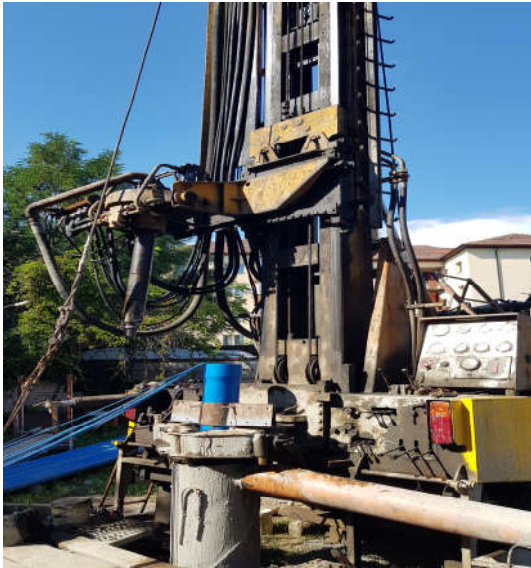
Figure 3. Drilling rig - T_{PVC} mounting
