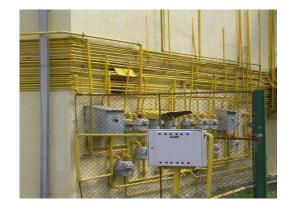
Figure 3. Gas network - pressure adjustment and measurement block
